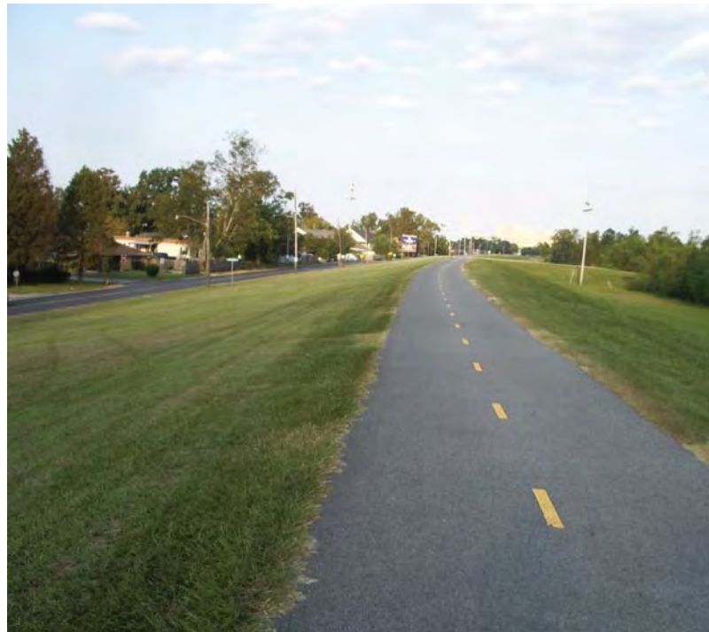
St. Charles Parish Multi-Use Levee Trail (East Bank)
