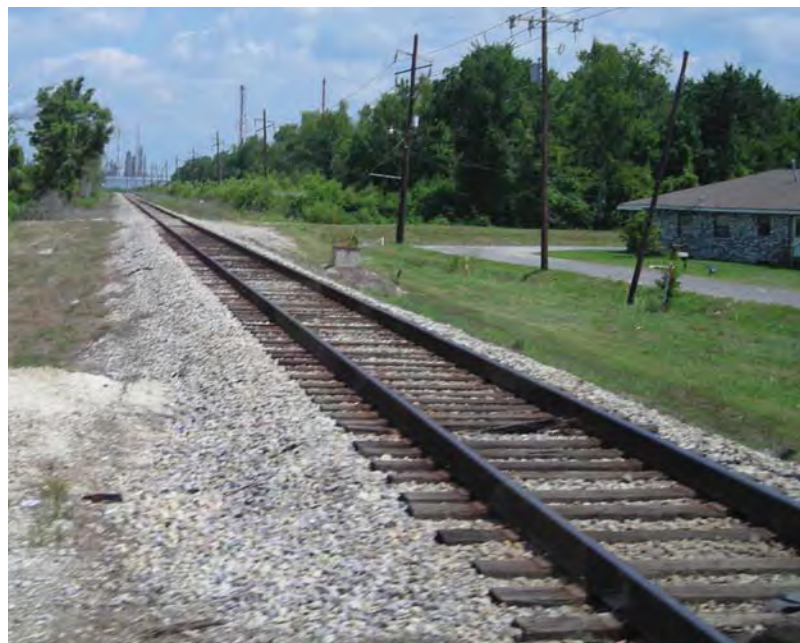
Union Pacific line, looking east from Ashton Plantation Blvd.
