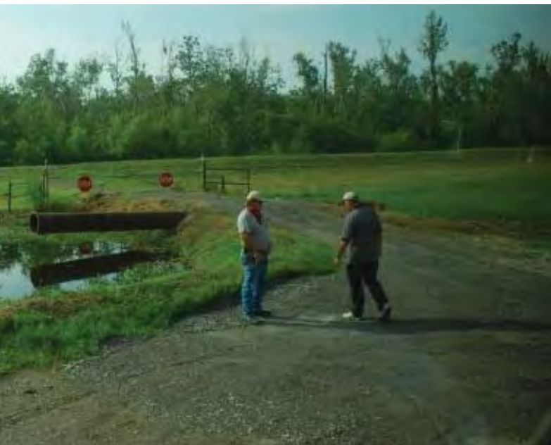
Levee at Magnolia Ridge
