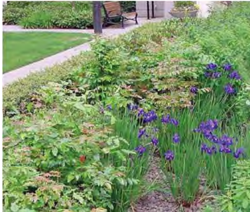
Best management practice for filtering runoff: vegetated swales
