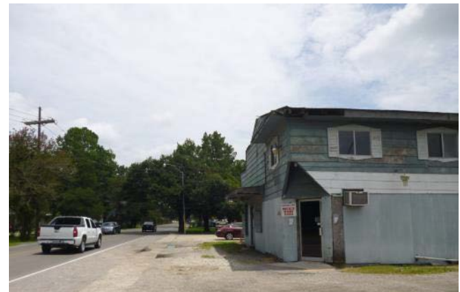
Existing commercial buildings on Paul Maillard Rd, Boutte
