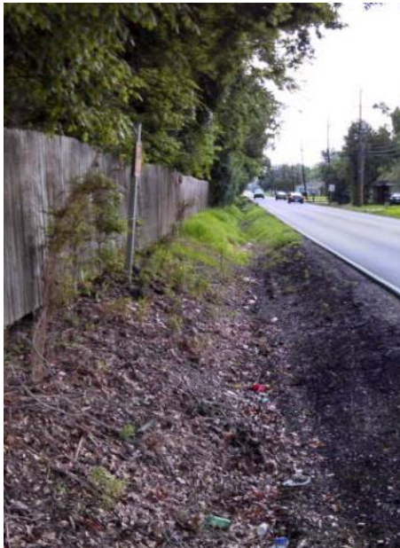
Open ditch along Paul Maillard Rd
