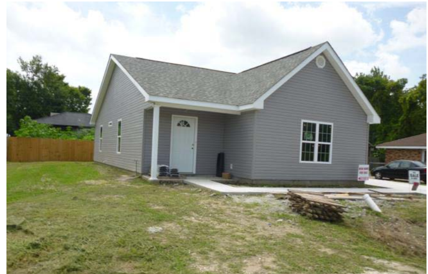
Example of residential infill, S. Kinler Street, Luling
