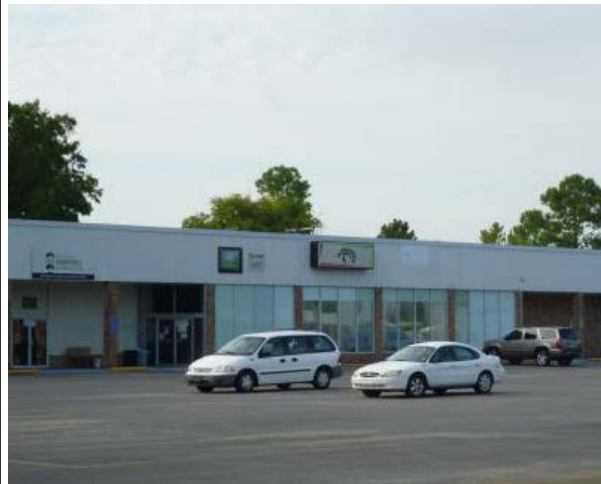
Louisiana WIA Offices, Paul Maillard Road
