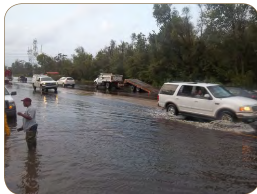
Flooding across US Hwy 61
