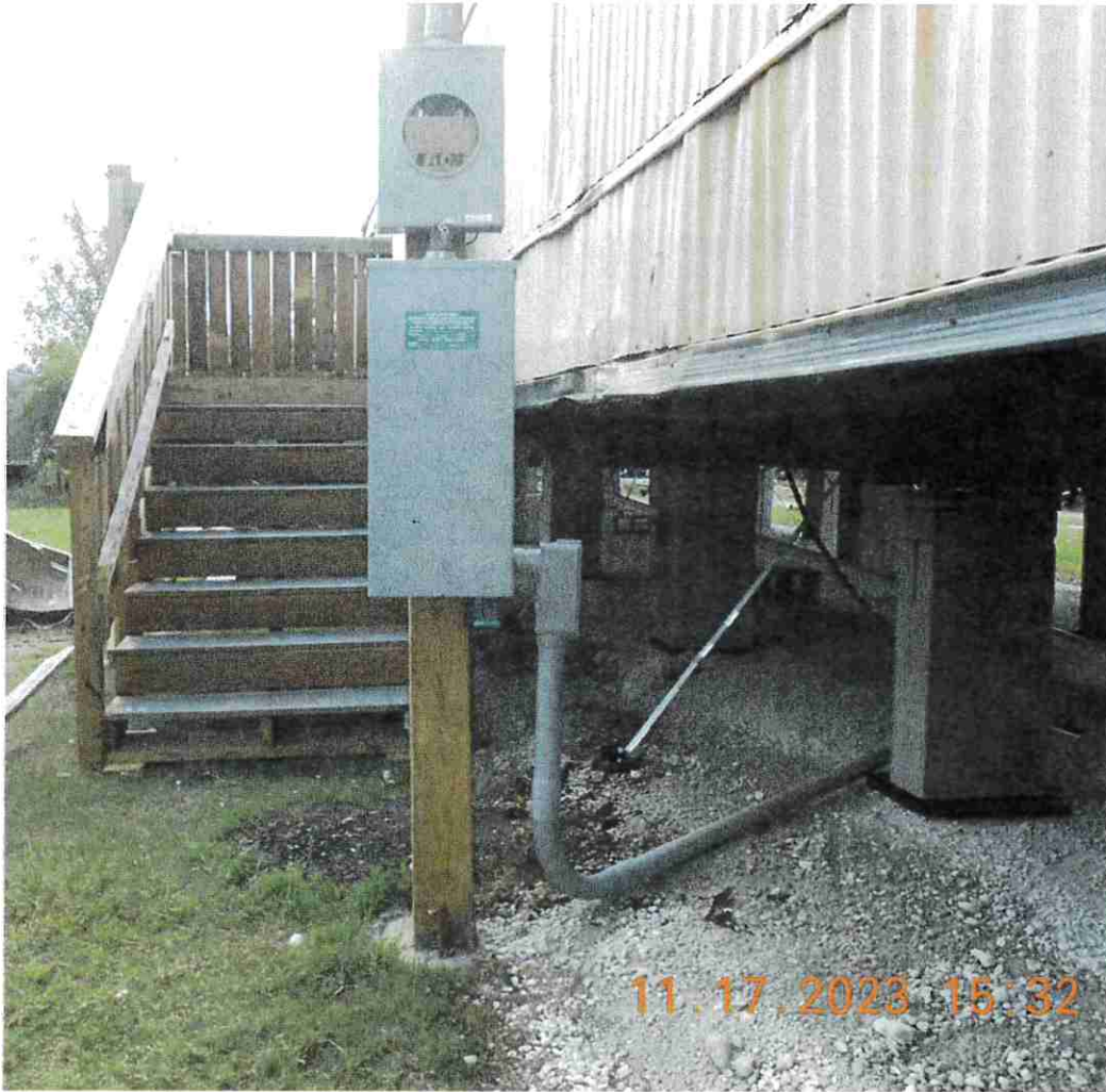
C2.e) Lowest machinery serving building is electrical panel located near front right corner of home.
